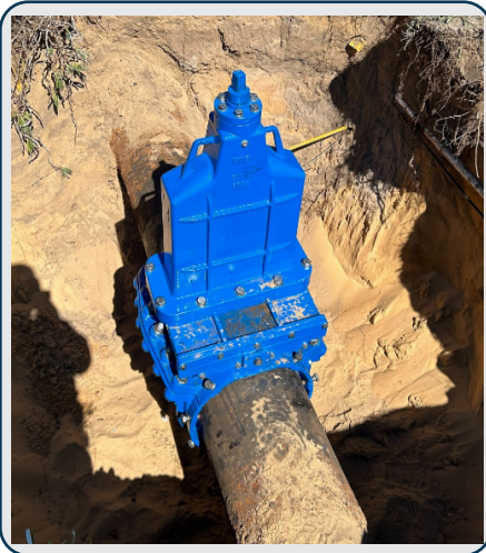
DN375 to DN500mm Novus Valve
